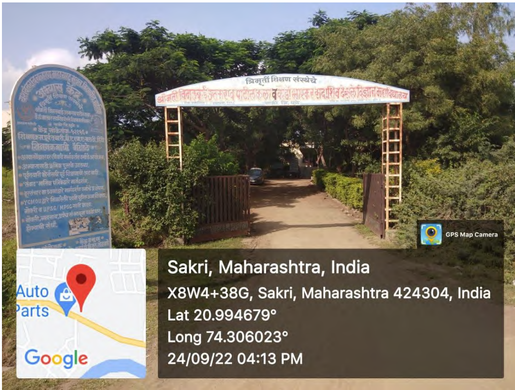
Photo 1 College campus main Entrance gate with dense vegetation
