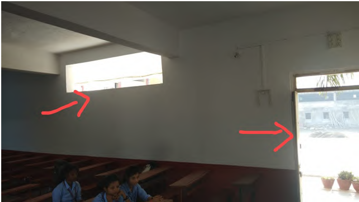
Photo 22 Classrooms of the college Campus are Well Ventilated, with a very good Window Floor ratio.
